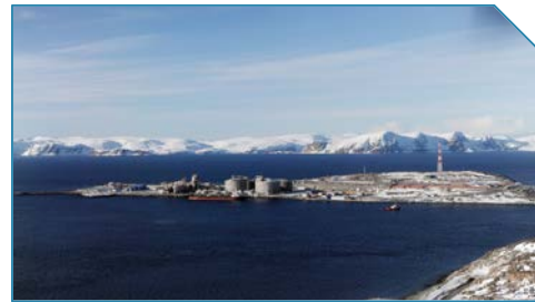
Nexans contribution to the Snøhvit gas field in the Barents Sea, largest ever industrial project in North Norway
