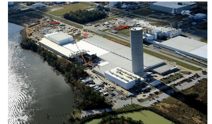
Charleston plant conversion delivery on track for Q3; Seagreen project manufacturing ongoing
